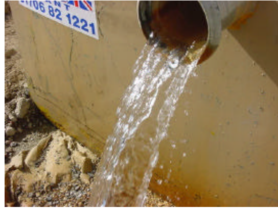
Water discharge from tank to trench
