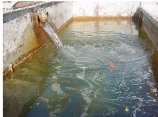
Water received at open settling tank
