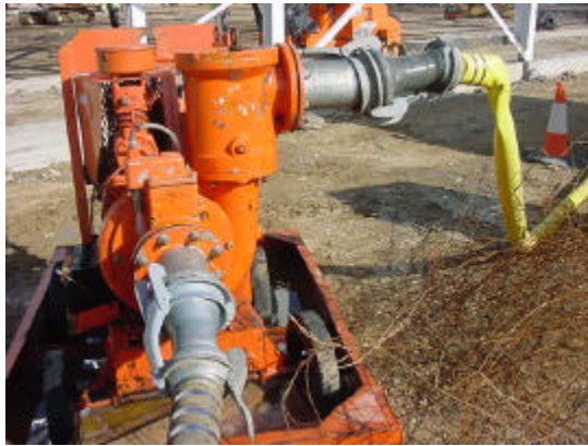
Pumping from trench
