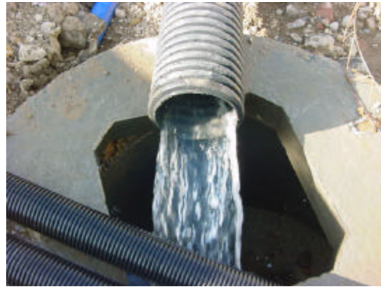
Discharge to site drainage
